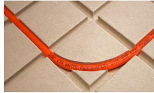
4. Test fit the path with a section of pipe before attaching the panel to the subfloor.
