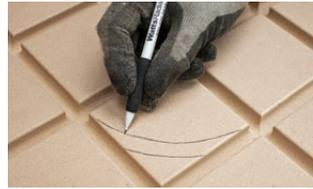
1. Trace the outline of a gentle curve using a length of pipe or a curve template.
